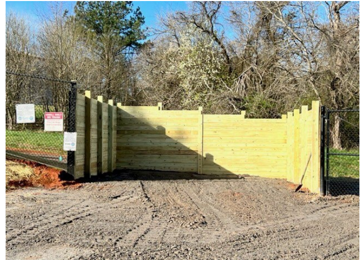
Figure 1: Upgraded public drop-off bin located in Greenville, SC Renewable Water Resources Facility
