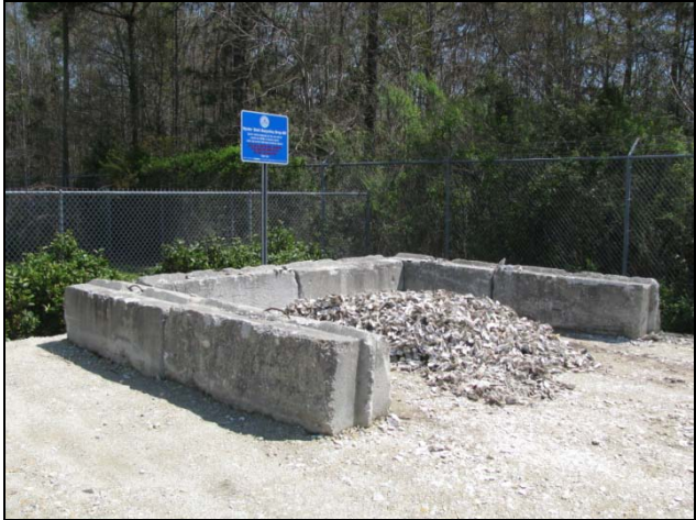
SCDNR has received positive feedback from local officials and the public for utilizing concrete barriers to create oyster shell recycling bins, due to their ease of maintenance.
